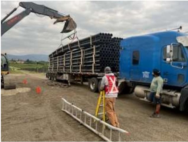
(truckload of 10 inch main pipe for irrigation project)
